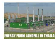
ENERGY FROM LANDFILL IN THAILAND
